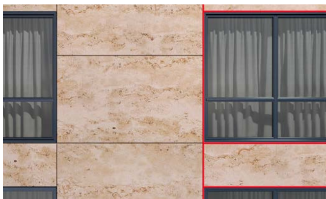
Joints in the facade area
