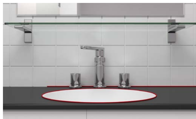
Connection joints in the bathroom
